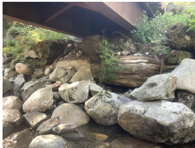
Left Bank Abutment when facing downstream
