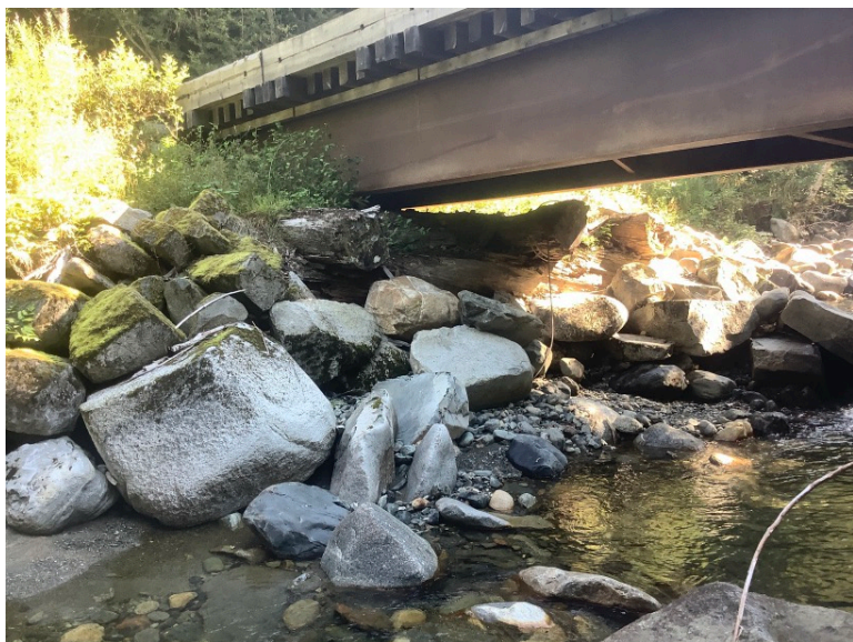
Right Bank Abutment when facing downstream
